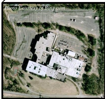
Figure 3 | Close-up Aerial View of Site
