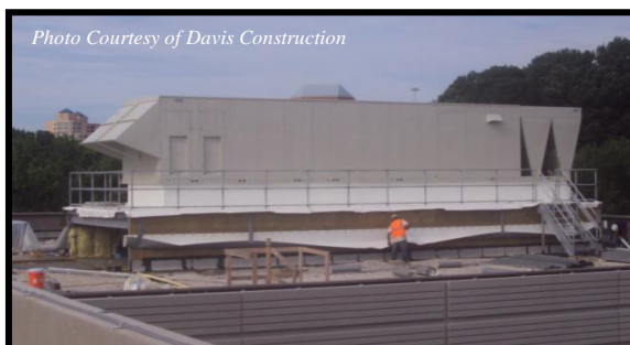
Figure 30: Roof top Air Handling Units
