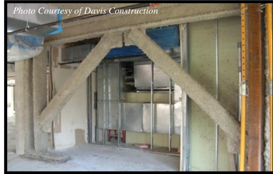
Figure 7 | Installed Seismic Bracing
