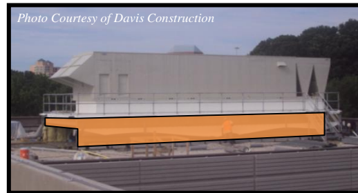
Figure 25 | Raised Platform for RTU
