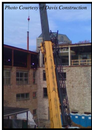
Photo Courtesy of Davis Construction Figure 32 | Installation of Progressive Collapse Steel System
