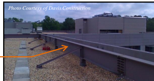
Figure 13 | Progressive Collapse Steel System Installed
